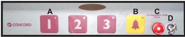
Figure 1 3 Stop COP Panel
